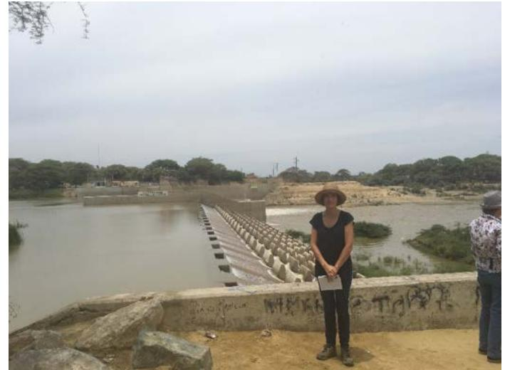
Piura, Peru: The Ejidos diversion dam serves to divert water for irrigation and flood control management just upstream of the city of Piura in Northern Peru, especially during El Niño events. (Photo of Martha Bell)
